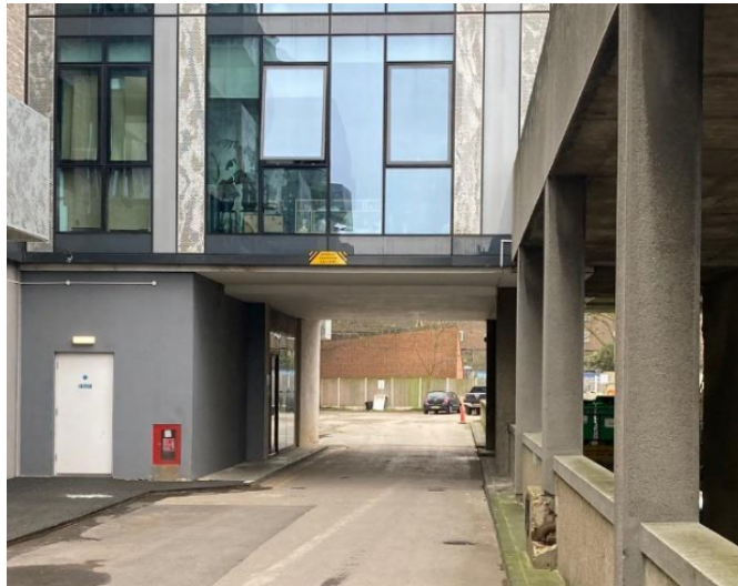
Image 7. Photo of rear servicing yard. The ground floor reception is on the left and the refuse/recycling store on the right.
