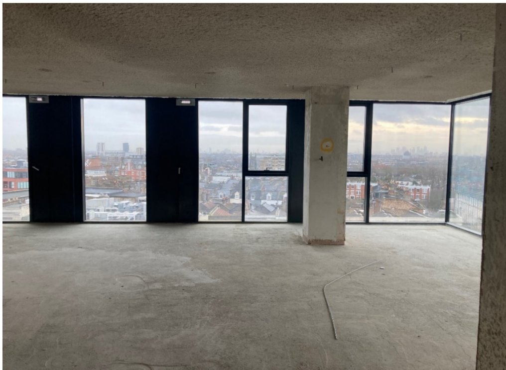
Image 2. Photos inside of the 6 th floor of Hill House.
