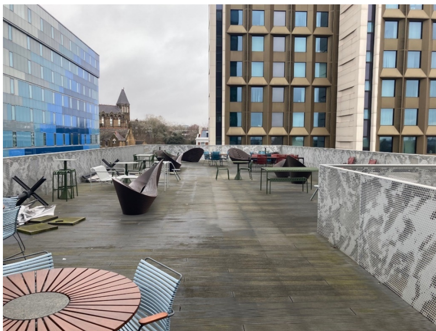
Image 3. Photo of existing communal roof terrace at 4 th floor level.
